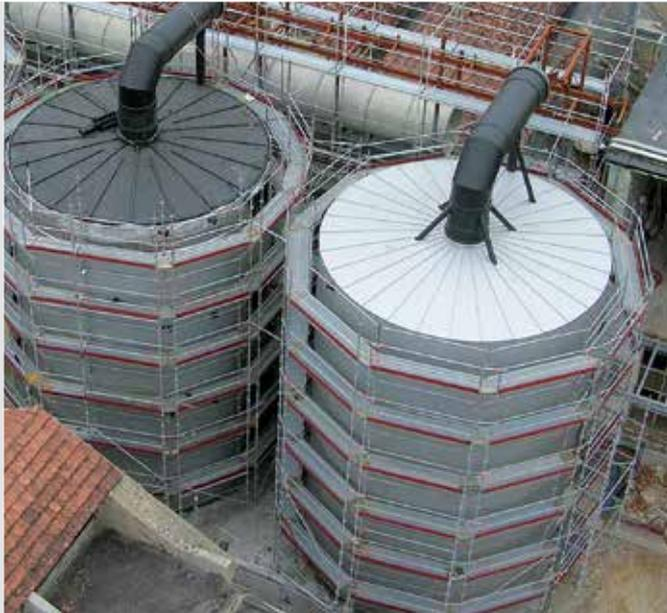
Air purification system, Spain. Material: HD-PE
