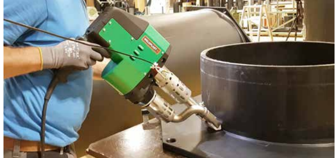
The powerful WELDPLAST S4 in use
